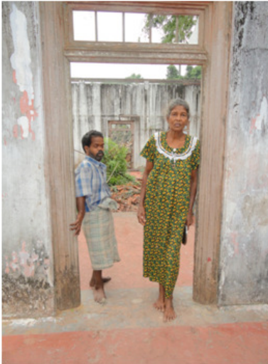
A widow (right) and her mentally disabled son, living in an abandoned roofless house.
