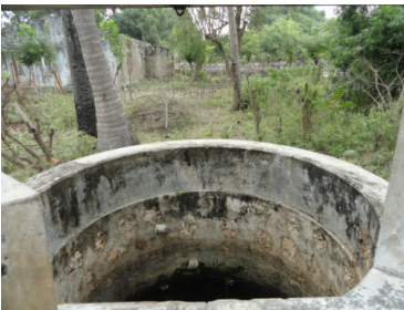
Unusable well in premises of the house occupied by displaced family.
